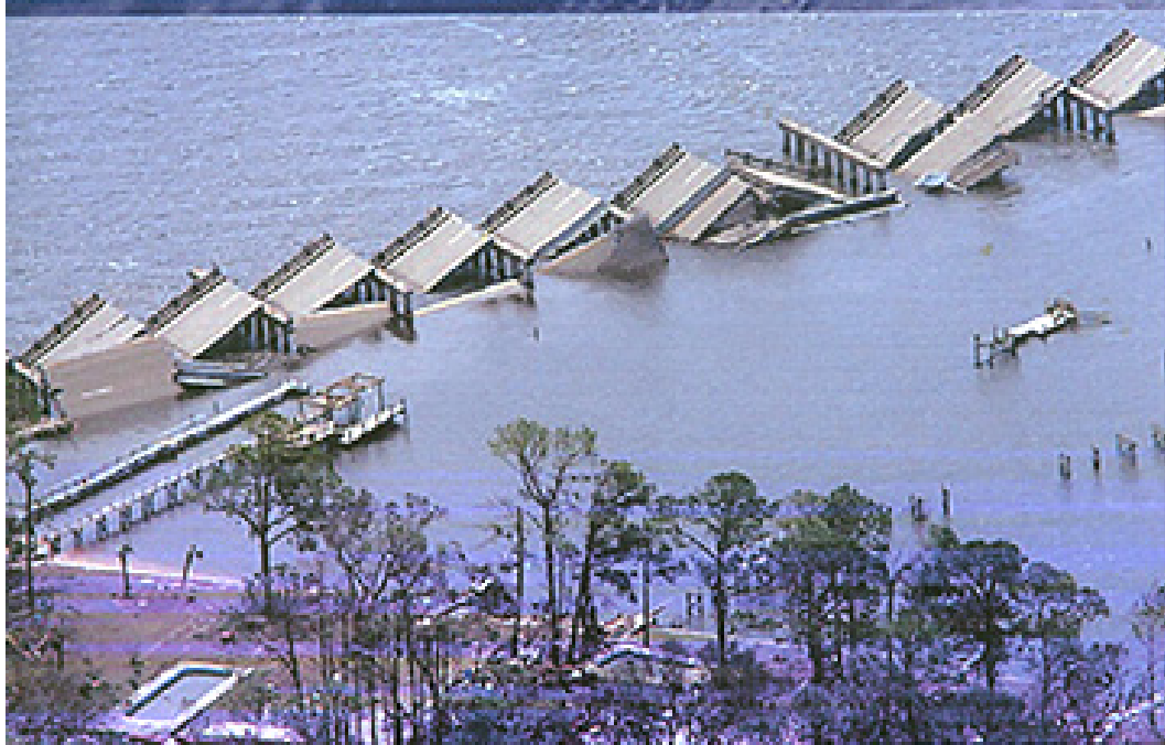
Figure 4.4 Hurricane Katrina damage to U.S. Highway 90 at Bay St. Louis, MS. (Source: NASA Remote Sensing Tutorial)
