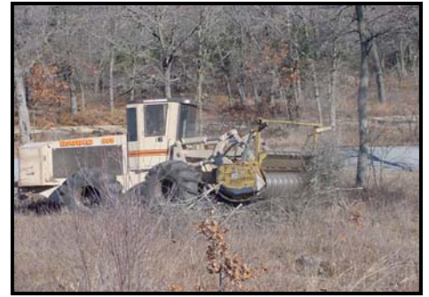
Removing brush and briars using a severe-duty shredder.
