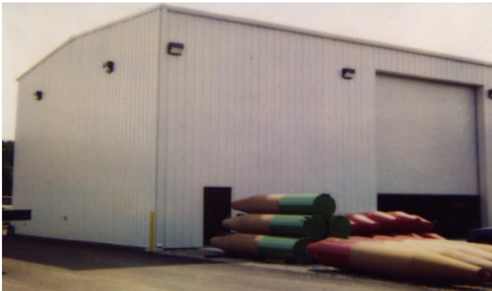
Addition to Buoy Depot, Support Center Boston: $215,000
