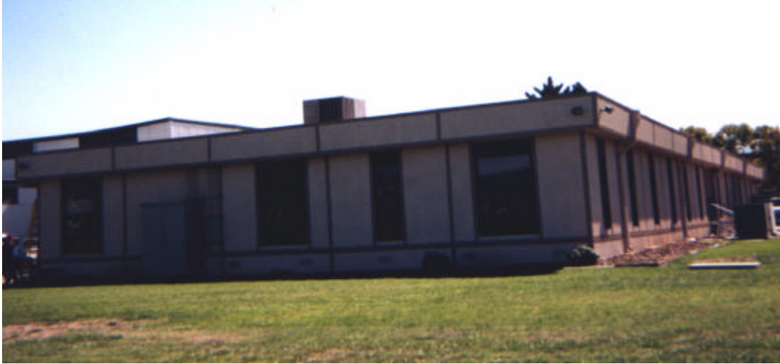
Modular Office Complex, Alameda, California: $811,000
