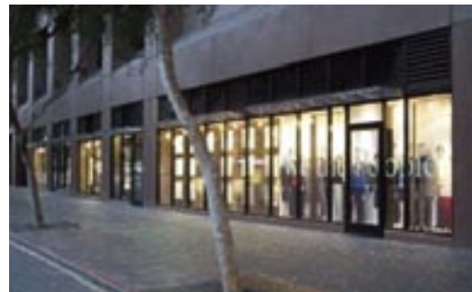
Edward J. Schwartz Federal Building, San Diego, CA, before (top) and after.
