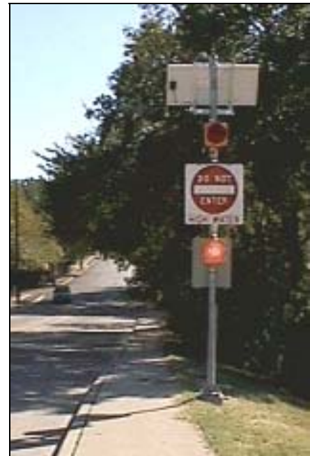
City of Dallas, TX Flood Warning System Sign Assembly
