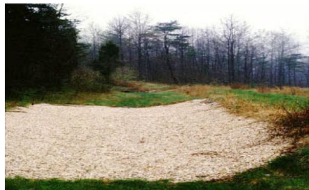
**Infiltration trenches allow stormwater to percolate slowly into the soil.**
