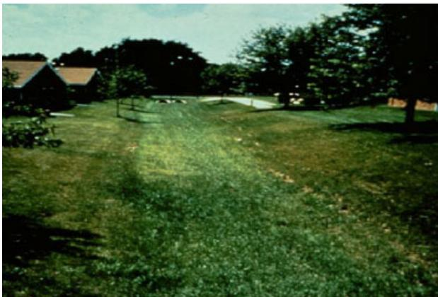
Grassed channels are effectively used along roadways to convey and infiltrate stormwater.
