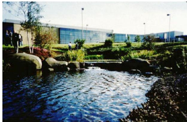
**Stormwater wet ponds are characterized by a permanent pool of water.**
