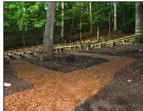
Treated engineered wood fiber improves routes and wheelchair spaces at an outdoor arena at Wolf Trap.
