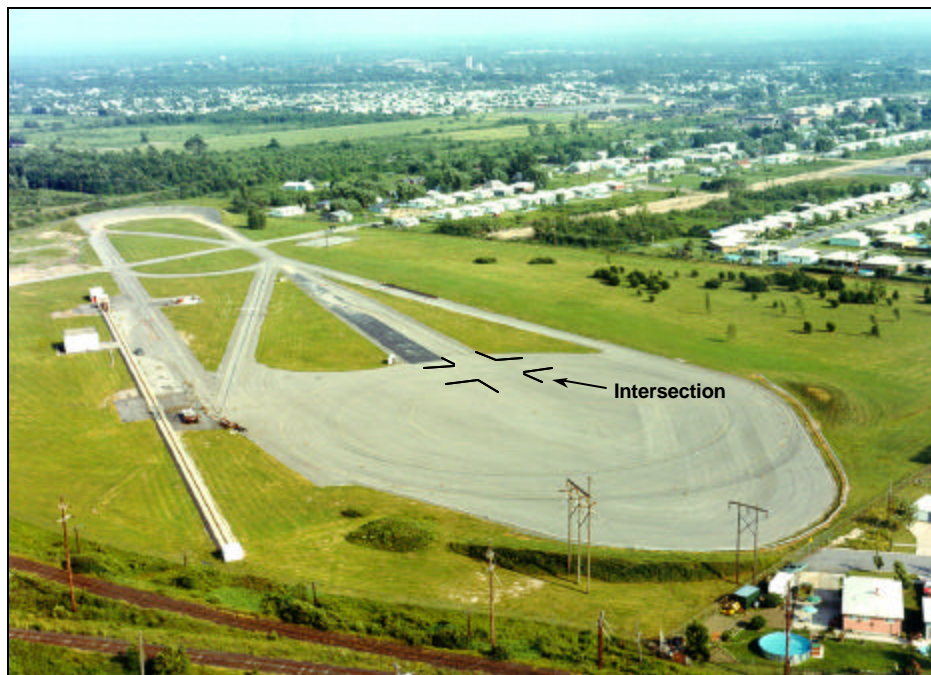
Figure 5-9 Veridian Test Track Facility
