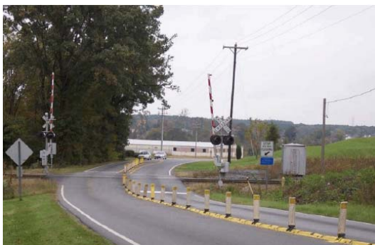
FRA supports use of channelization devices to deter motorists from driving around lowered gates at highway-rail grade crossings.
