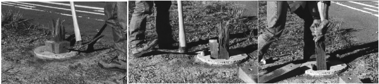
Removing broken signpost from quick install location
