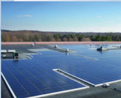
Janssen Pharmaceutica’s solar photovoltaics array was the third largest in the United States at the time of installation (2003).
