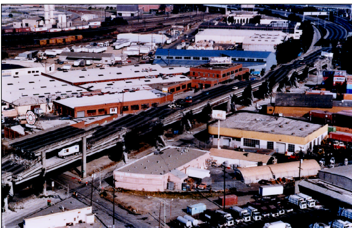
The 1989 Loma Prieta earthquake damaged the Cypress Freeway beyond repair.
