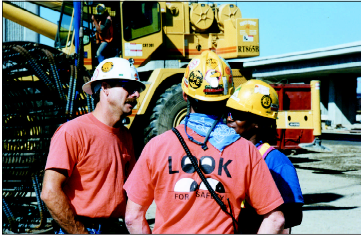
Caltrans financed the Cypress/Mandela Training Center to provide Oakland residents with skills necessary to participate in the freeway reconstruction project.
