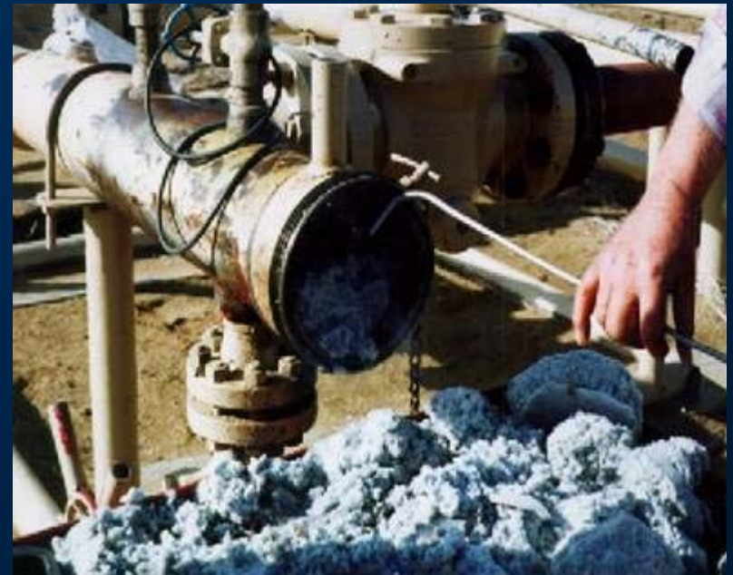
Methane hydrates blockages
