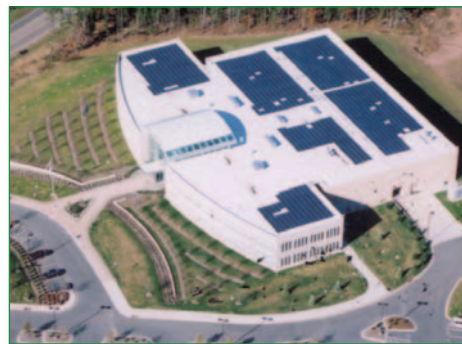
The roof of EPA's computer center in RTP, NC, is covered with solar panels.
