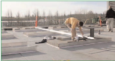
Workers install the PV roof at EPA's Oregon facility.
