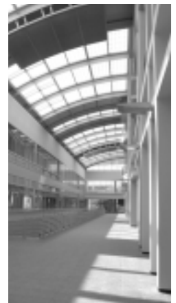
The atrium provides daylighting and improved thermal insulation.
