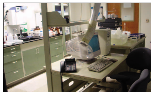
To save energy and reduce air flow, 18 articulated snorkel exhaust hoods were removed during a recommissioning project at EPA's NEIC laboratory.
