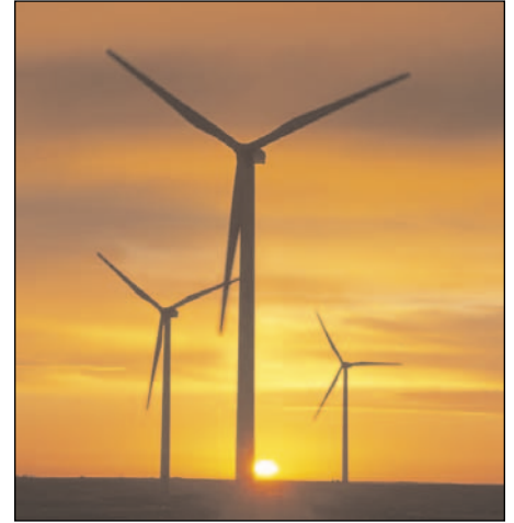
Recent green power purchases for five EPA facilities support wind power projects such as the Edgeley/Kulm wind power project in North Dakota.
