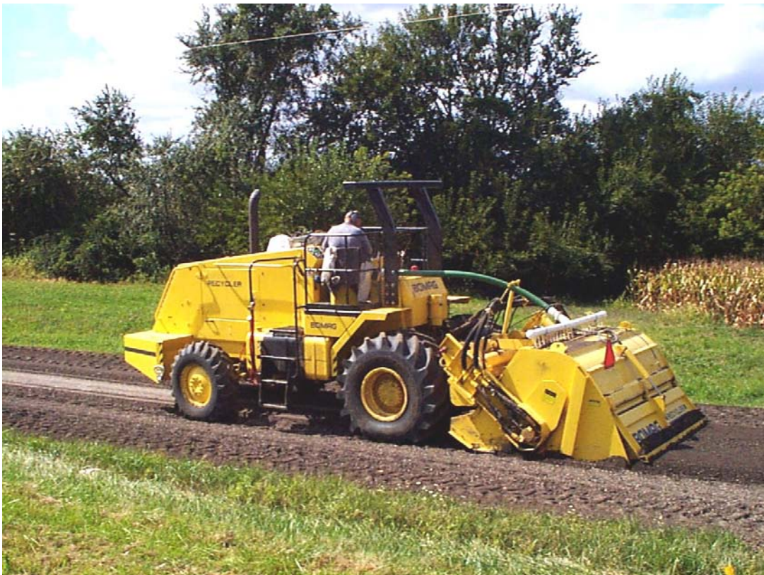
Figure 8-16. Roadway stabilizer/mixer (photo courtesy of Bomag).
