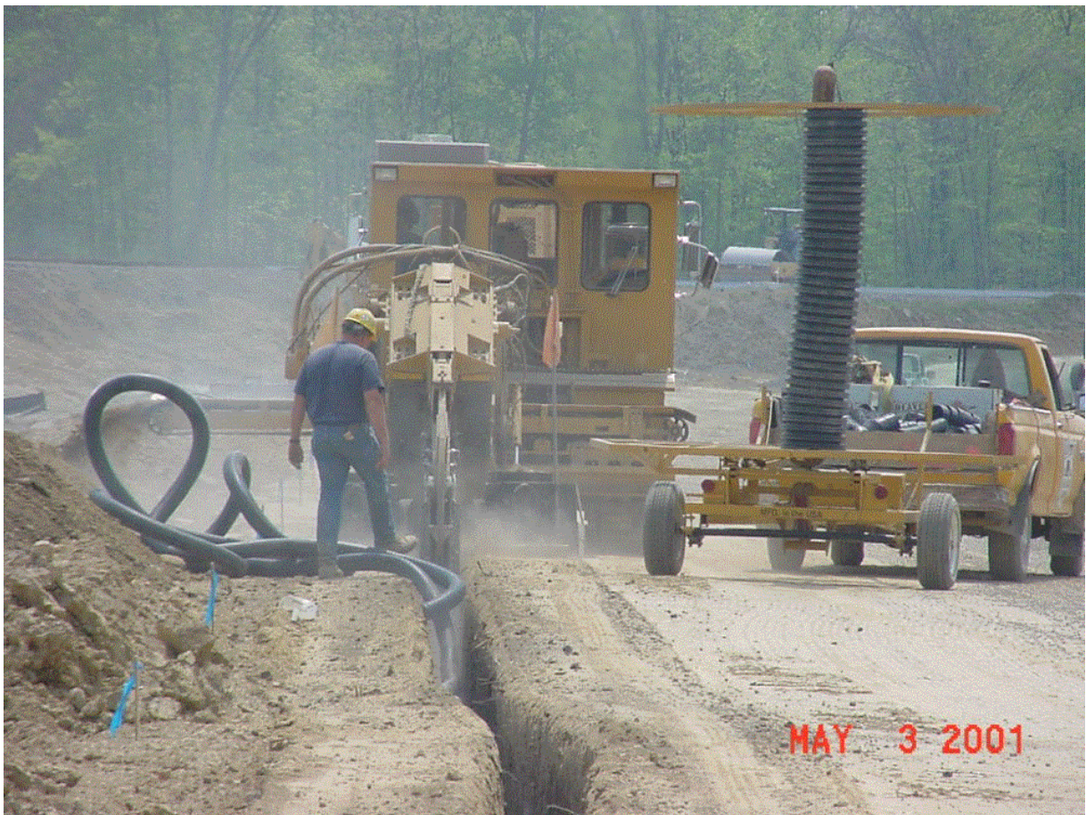
Figure 8-4. Underdrain installation ( photo courtesy of Ohio DOT ).
