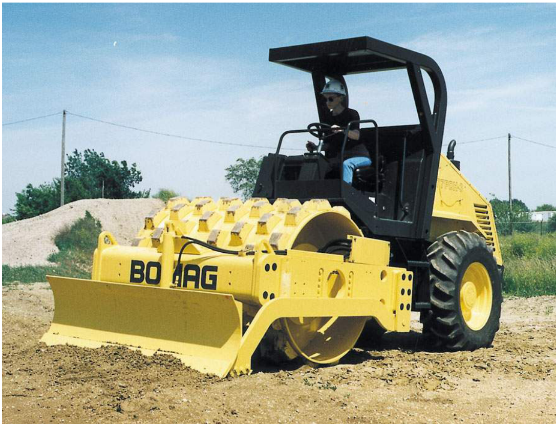
Figure 8-13. Sheepfoot roller ( photo courtesy of Bomag ).
