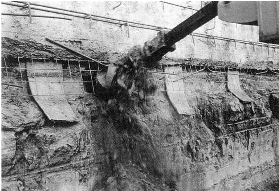
Figure 4.5: Strip Drains under Temporary Shotcrete.
