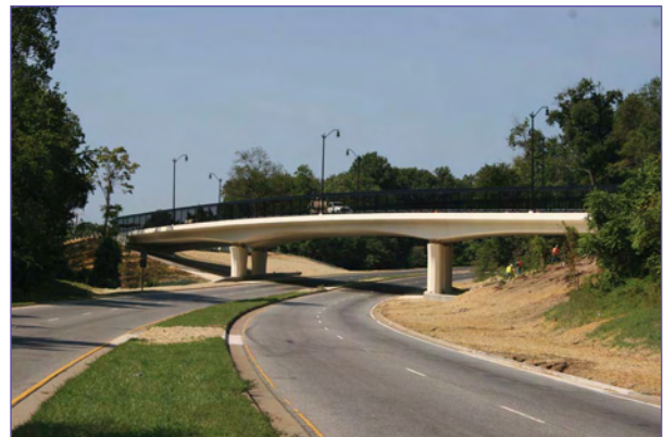
After—Southern Avenue Bridge Project Replacement, Washington, District of Columbia (District Department of Transportation)
