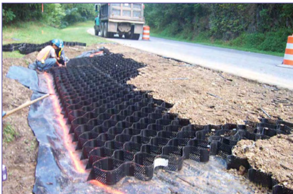
Placement of Geoweb—Green Parking Area Alternative, Great Smoky Mountains National Park, Tennessee (National Park Service)
