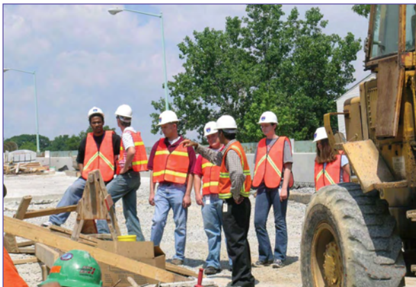
Co-op students at Taylor Street Bridge Replacement, DC BH-3202(8), Washington, District of Columbia (District Department of Transportation)
