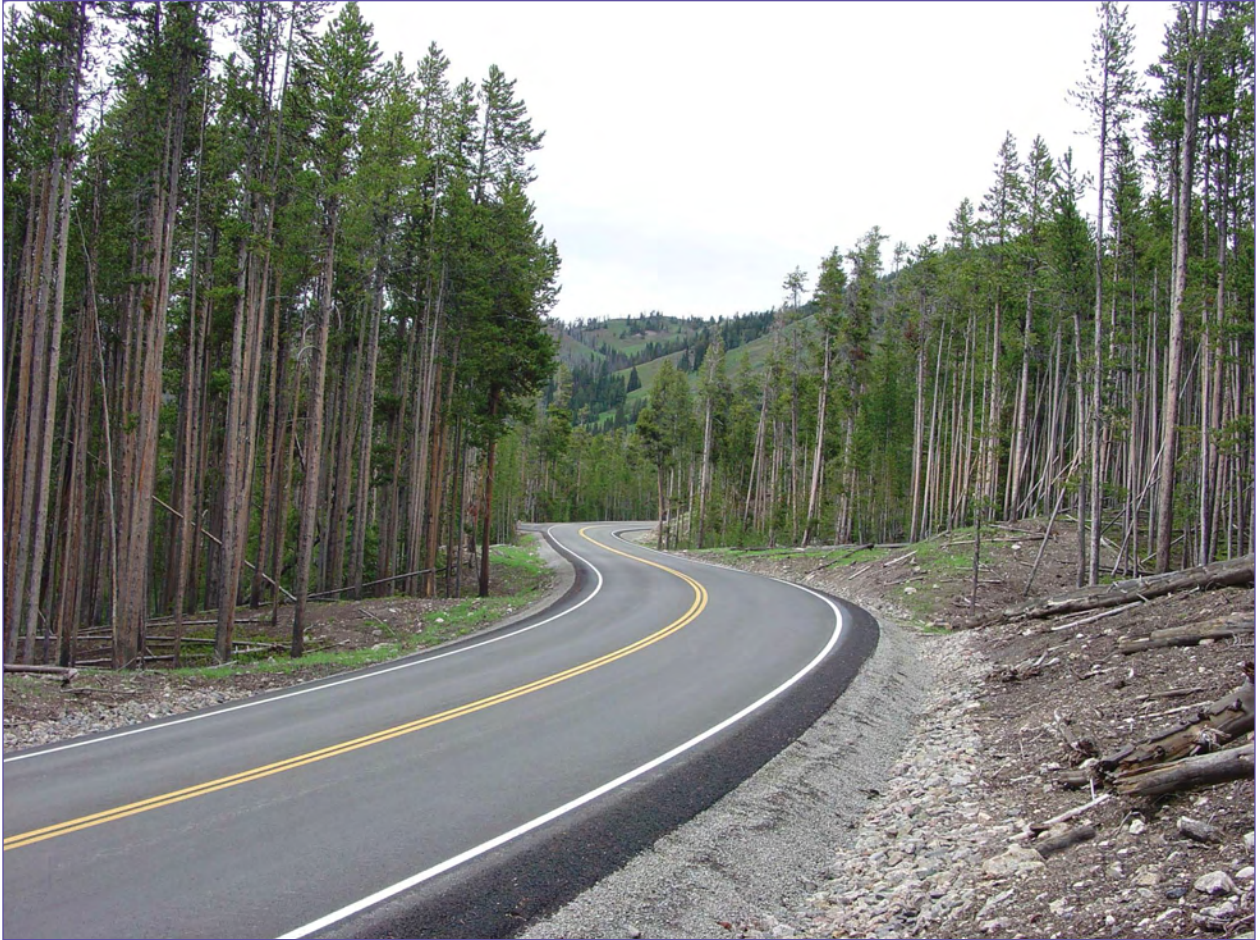
Grand Loop Road, Yellowstone National Park, Montana (National Park Service)
