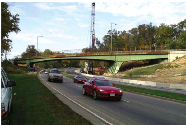
Before—Southern Avenue Bridge Project Replacement, Washington, District of Columbia (District Department of Transportation)
