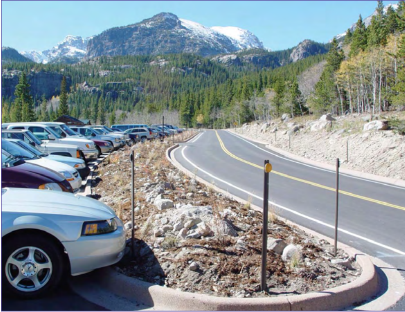
Relocation of parking areas increases safety and decreases environmental impacts. Bear Lake Road, Rocky Mountain National Park, Colorado (National Park Service)
