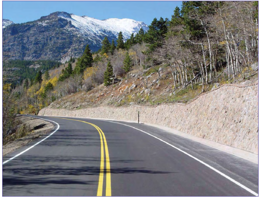
Use of real stone facing blends the retaining walls with the terrain. Bear Lake Road, Rocky Mountain National Park, Colorado (National Park Service)
