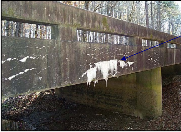
Figure 3. Cracking and efflorescence forms stalactites along the underside of the center span.
