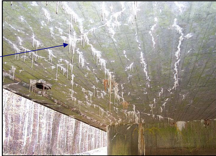
Figure 3. Cracking and efflorescence forms stalactites along the underside of the center span.
