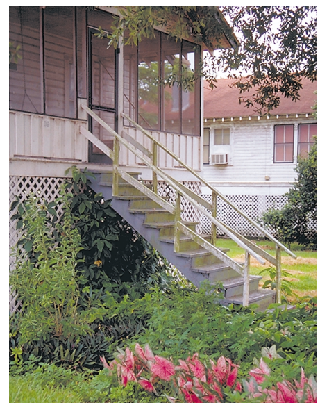
This building at the Everglades Experiment Station was originally constructed at the land surface; latticework and stairs were added after substantial land subsidence.
