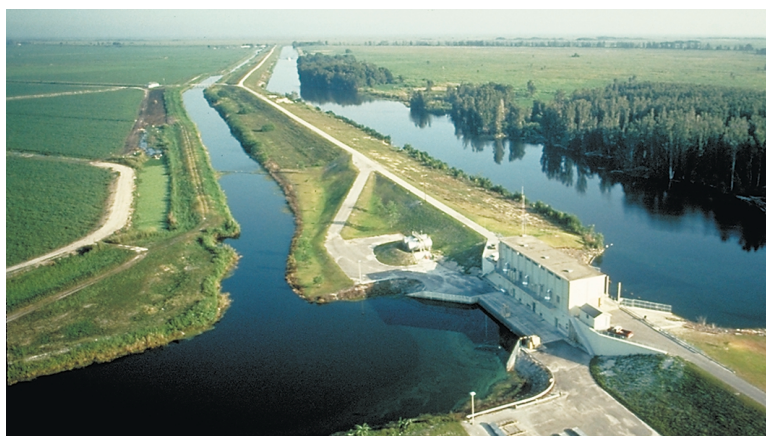
A network of dikes and canals controls water movement, providing optimum irrigation and drainage for sugar cane (left).
