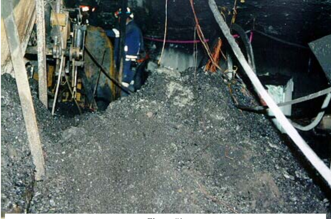
Figure #1 Coal Spill from Discharge Roller of #2-3NW Belt onto the #1-3NW Belt
