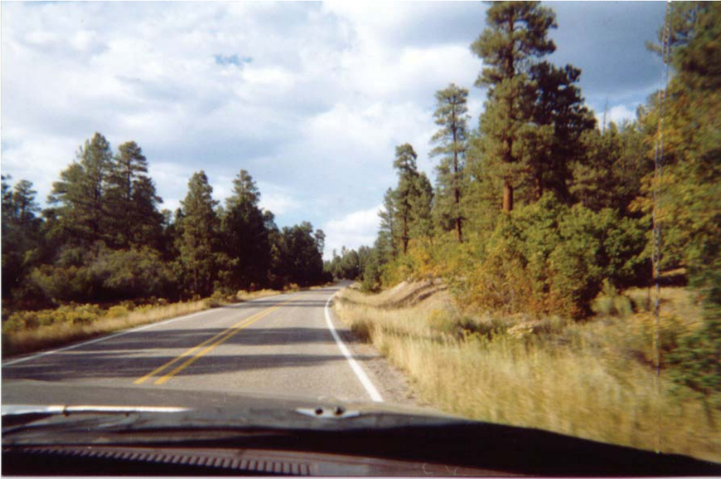
Figure 4. Photo. Representative wooded area traveling north on SR537.
