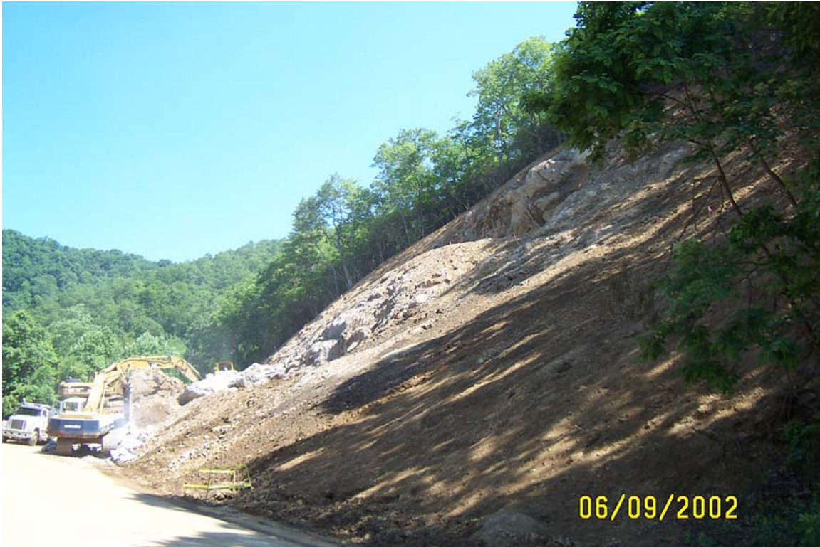
Excavated slope prior to the placement of the compost material.
