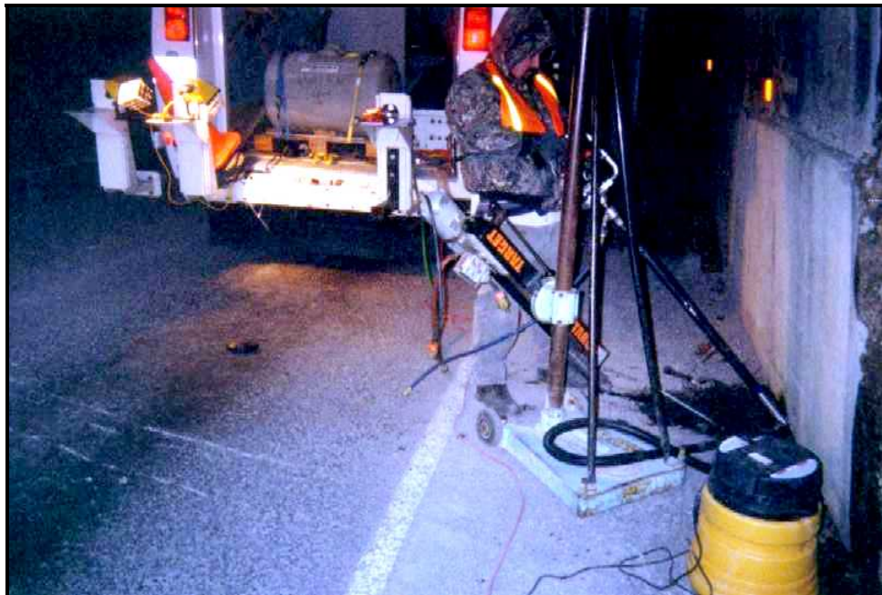
Figure 3. Coring equipment capable of drilling to more than two meters deep.
