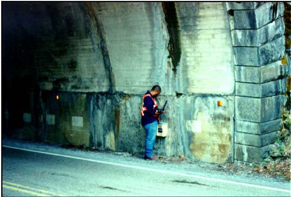
Figure 1. GPR antenna (top photograph) and survey in progress on the tunnel wall (bottom photograph).
