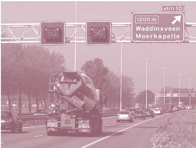
Figure 33. Congestion warning system in the Netherlands. (45)
