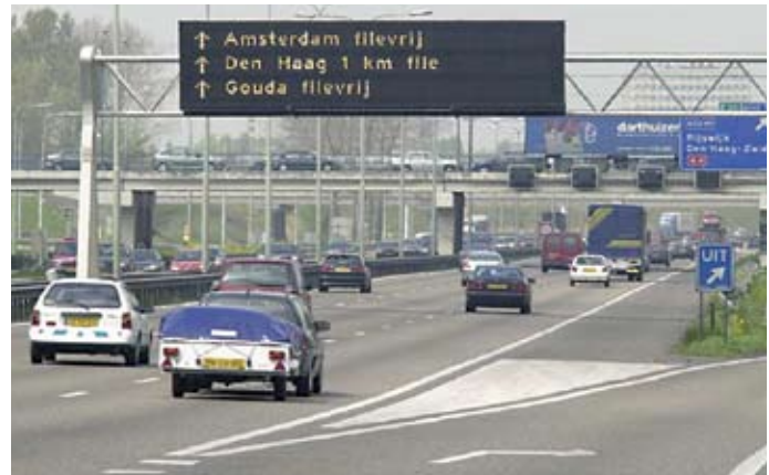
Figure 41. Dynamic route information panels in the Netherlands. (45)
