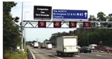
Figure 49. M42 ATM with hard shoulder running. (58)
