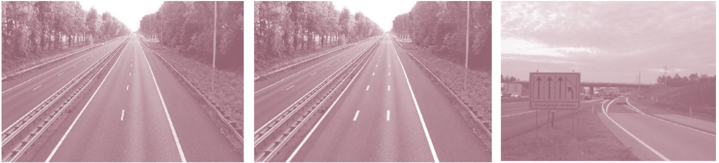
Figure 38. Dynamic lane marking in the Netherlands. (45,49)
