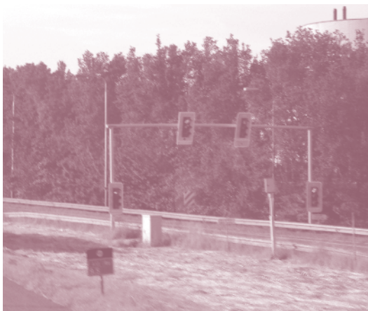
Figure 40. Ramp metering in the Netherlands.
