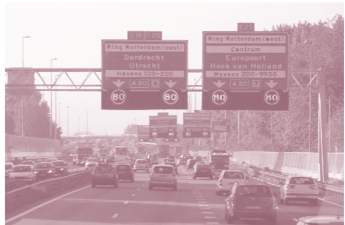
Figure 63. Variable speed limit displays in the Netherlands.
