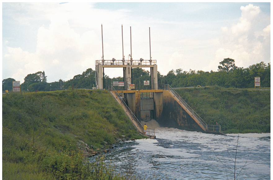
Figure 4. Structure S-49 along the C-24 Canal.
