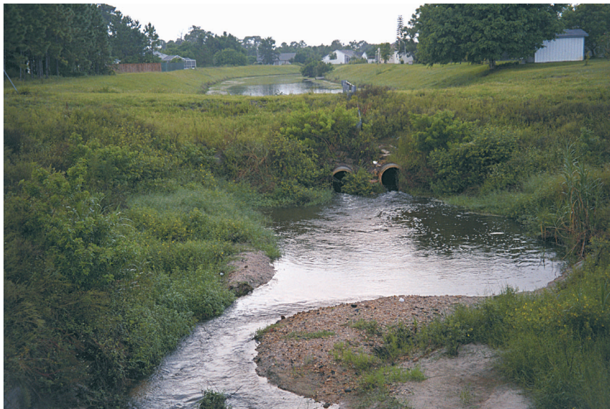
Figure 5. An inflow point to the C-24 Canal in an urban area.
