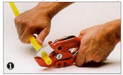
Cut the PE piping so that the end is square.
