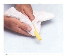
Clean pipe thoroughly to assure there is no dirt, grease or oil in assembly area. Also, assembly area must be free of severe scratches.
