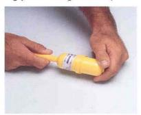
5 Stab pipe completely into fitting so that the mark on the pipe is flush or less from the fitting entrance.
