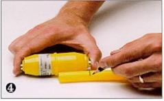
Use a soft felt pen, crayon or grease pencil to mark the stab depth as indicated on your Permasert package instructions. The stab depth is the approximate distance from the edge of the fusion bead to the end of the fitting body.
