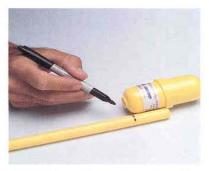
4 Holding the end of the pipe against the collar on the fitting, mark pipe at the entrance of the fitting (this stab length is 1 7/8").
