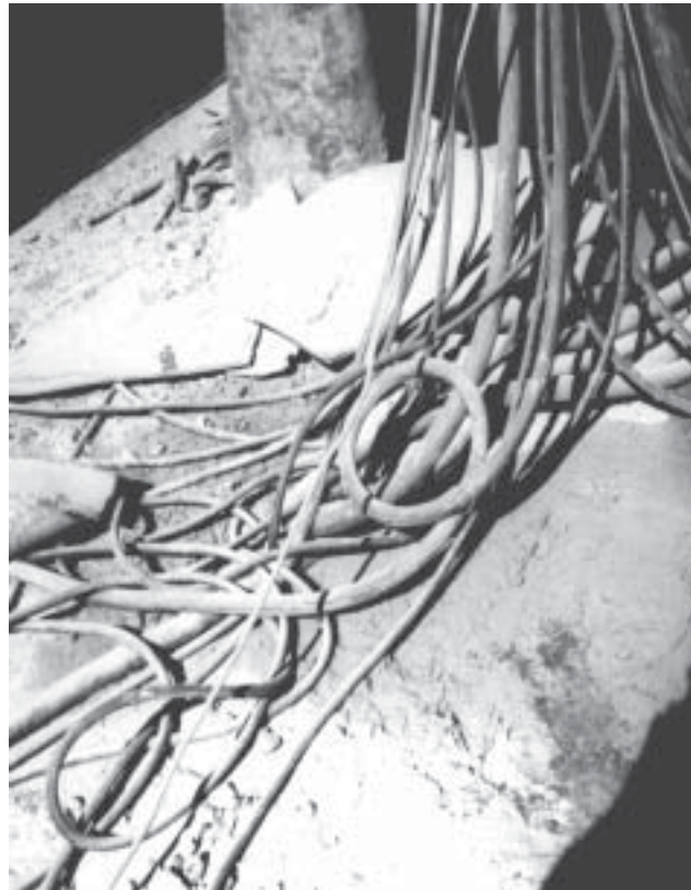
Unseen hazards for slips, trips and falls such as cables on the floor.
