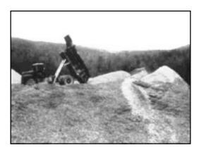
A good rule-of-thumb is to dump at least one truck-length back from the edge...
