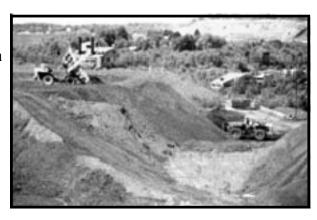
...then push the material over with a track-mounted dozer.
