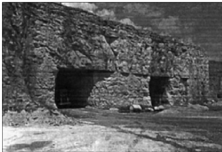
Figure 2.—A smooth roof line produced by a persistent bedding-plane lamination within the limestone roof beam.
