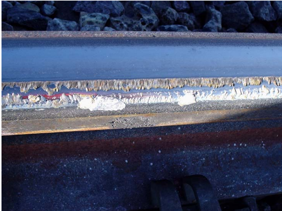
Figure 17. Laser-Treated Rail After 5.6 MGT Showing Two Spalls. Compare with Same Location as Shown in Figures 9 and 10 After 1.2 MGT
