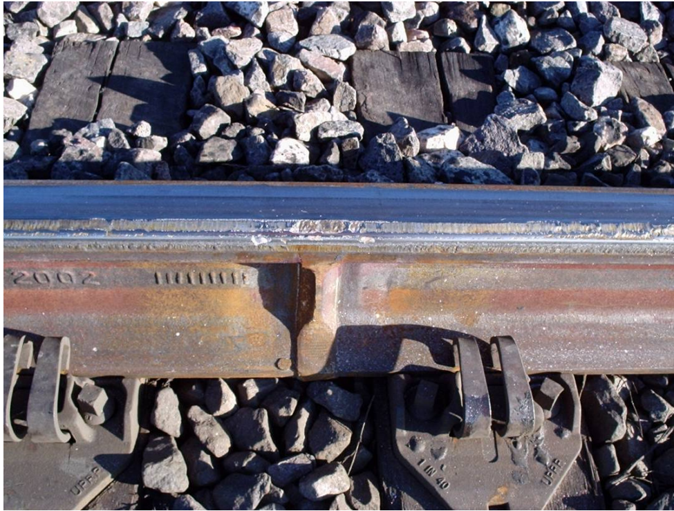
Figure 19. Thermite Weld on Laser-Treated Rail Segment After 5.6 MGT
