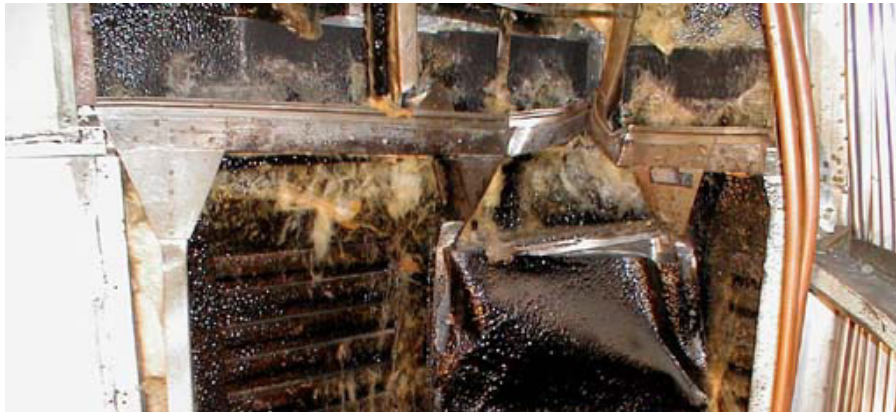
Figure 20. Left-side Cant Rail Between Window Frame (left) and Bulkhead Wall (right)
