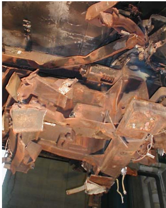
Figure B1-28. Forward Draft Sill - Right-side Deformations
