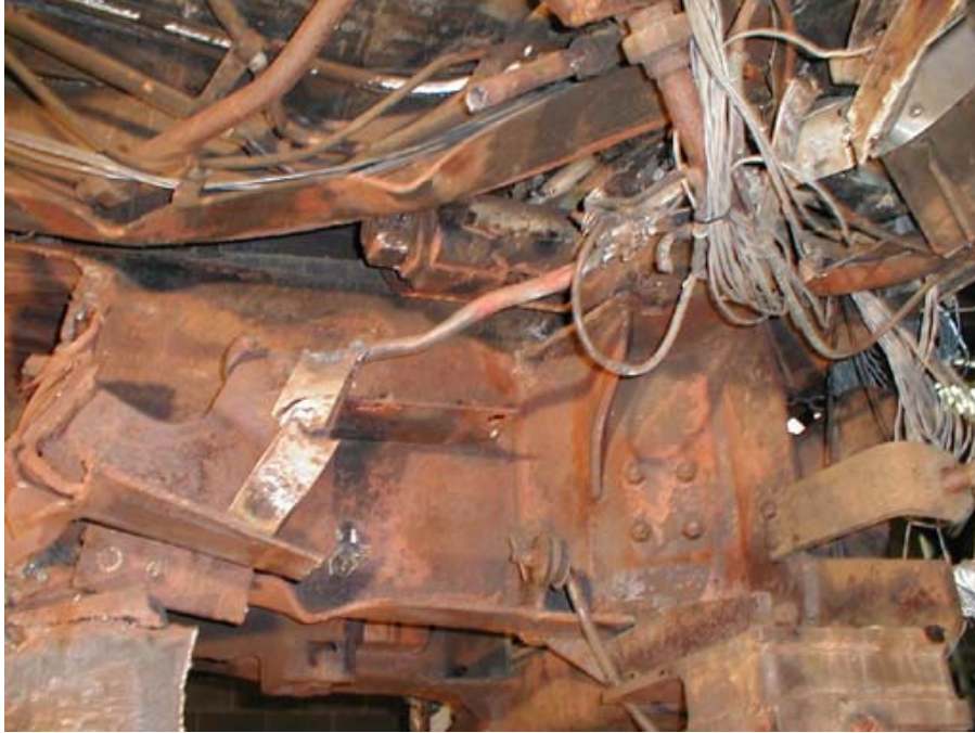
Figure B1-11. Forward Draft Sill, from Right Side Looking Slightly Upward
