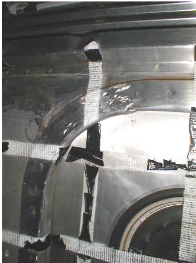
Figure B5-6. Buckle in Rain Gutter Above Top Left Corner of Right-Rear Door Frame
