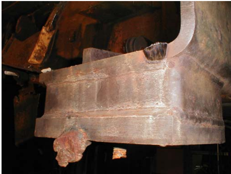
Figure B6-8. Wheel Burn on Lower Forward Draft Sill - Right Side
