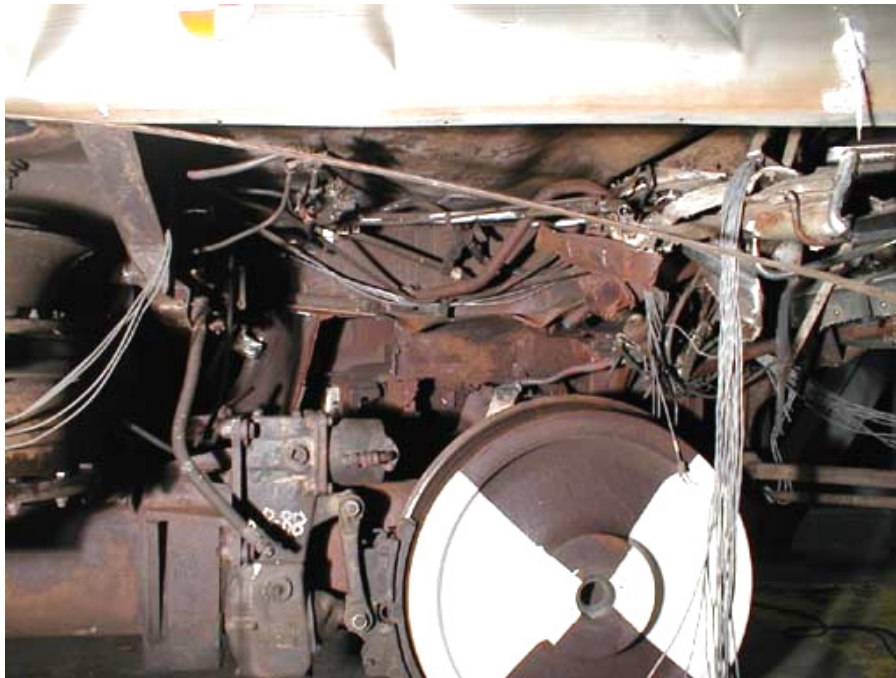
Figure B1-6. Right-side Draft Sill Collapse Before Truck Removal
