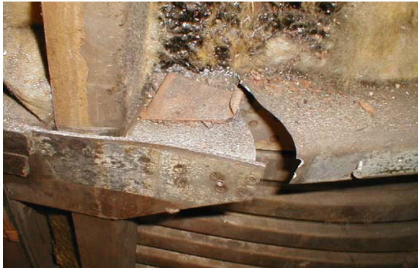
Figure 25. Left-side Belt Rail—Crack Detail Just Forward of Window Frame
