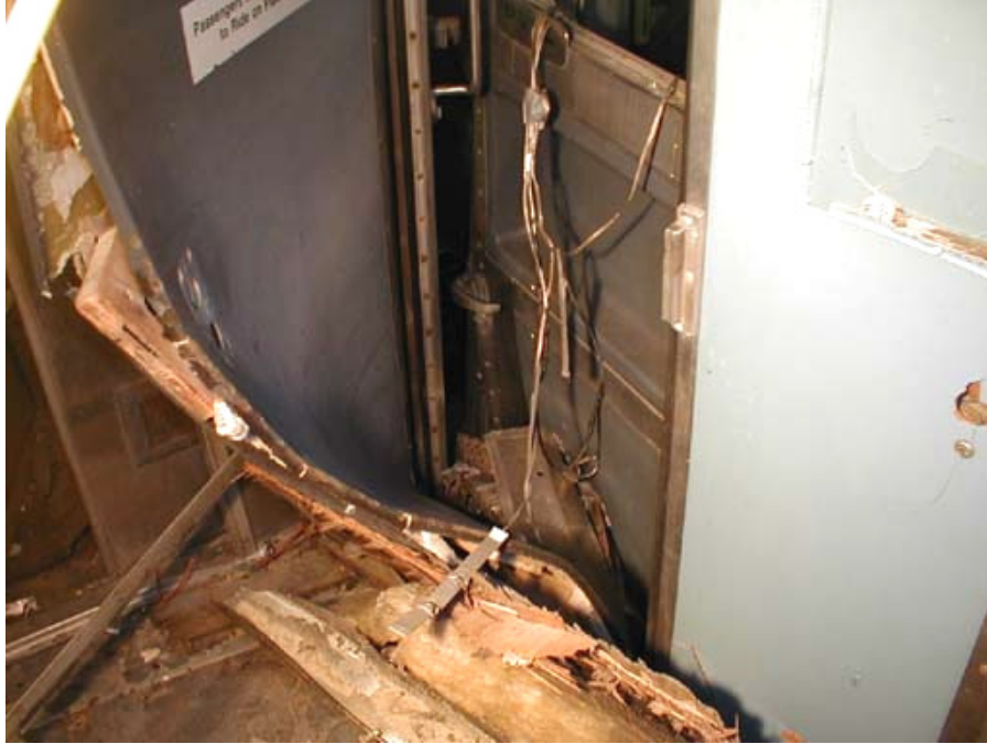
Figure B3-7. View From Inside of Vestibule Area Through Bulkhead Door
