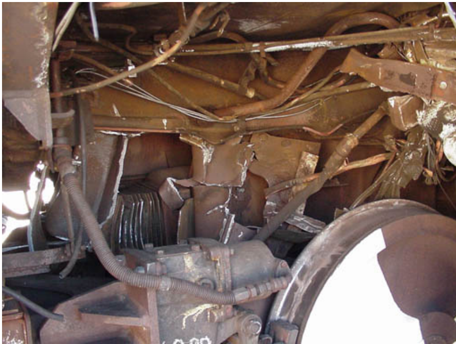
Figure B1-2. Right Side of Draft Sill Just After Test—Prior to Any Material Removal
