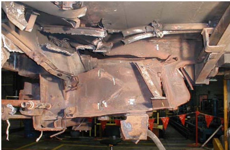
Figure B1-24. Left Side of Draft Sill After Material Removal
