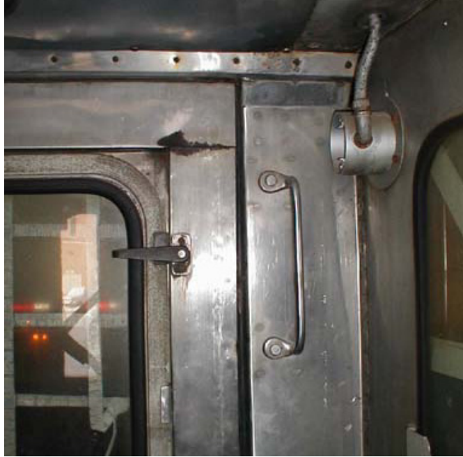
Figure B5-5. Detail - Door Frame Deformation in Right-Rear Door
