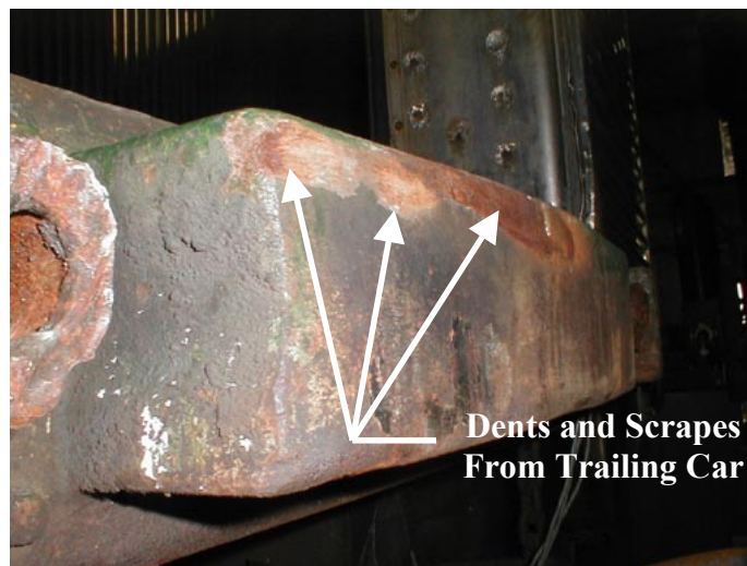
Figure 35. Evidence of B-End Impact on Buffer Beam
