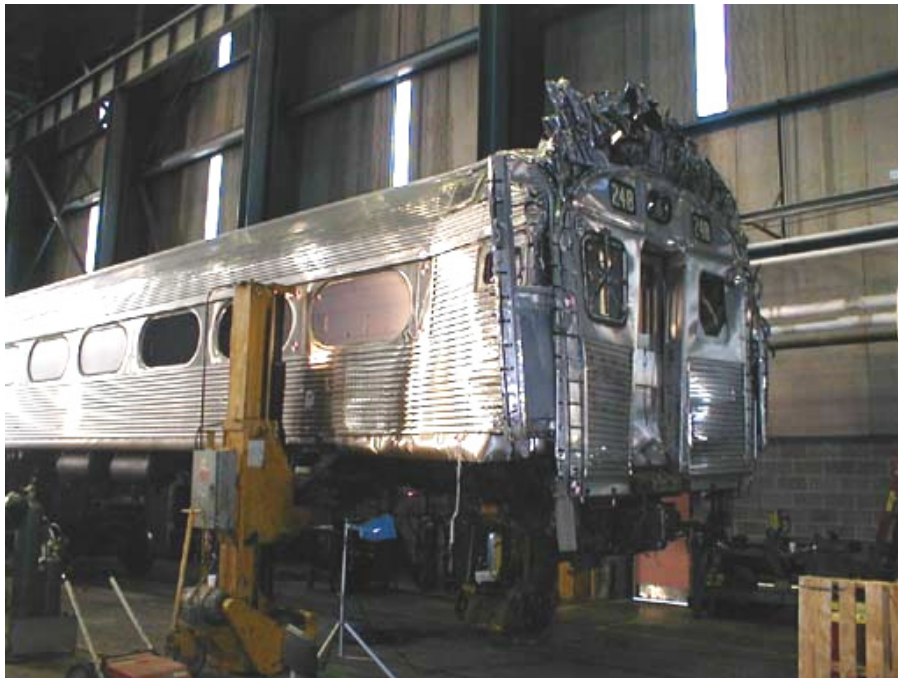
Figure B4-2. Right Front Corner of Damaged End—Car Jacked in Air in TTC RDL Building
