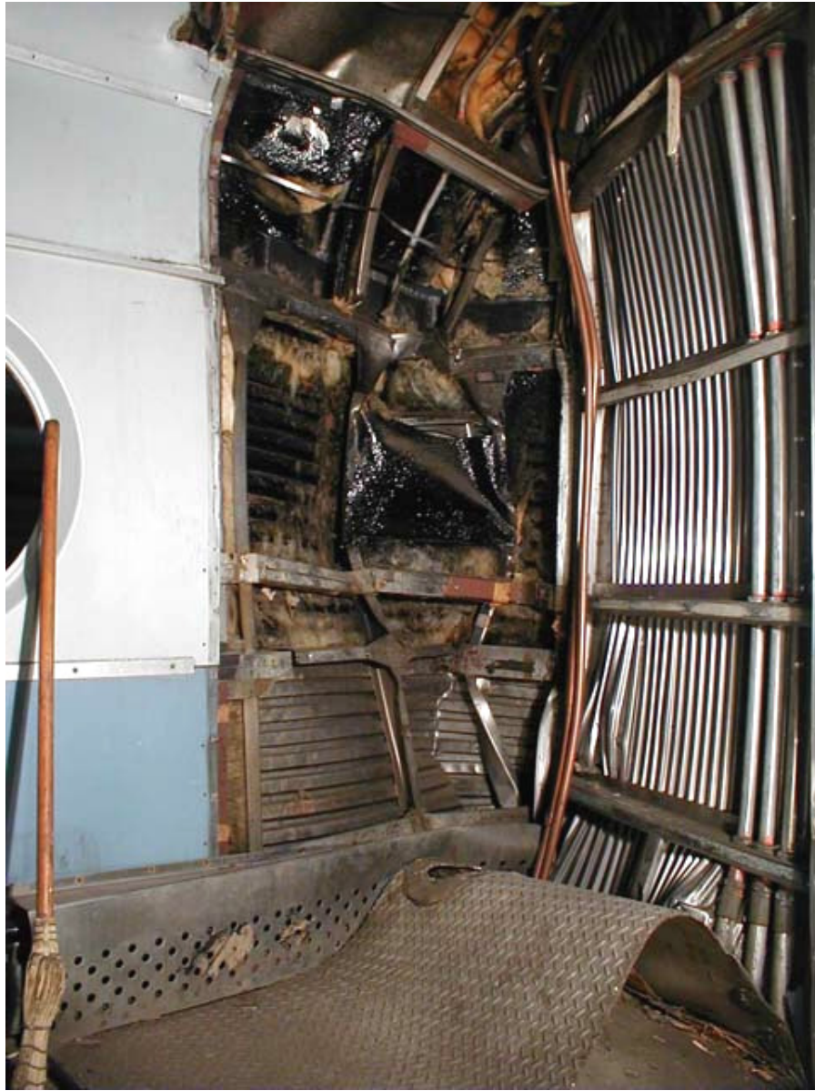
Figure B3-11. Left-side Front Corner Aft of Bulkhead Wall
