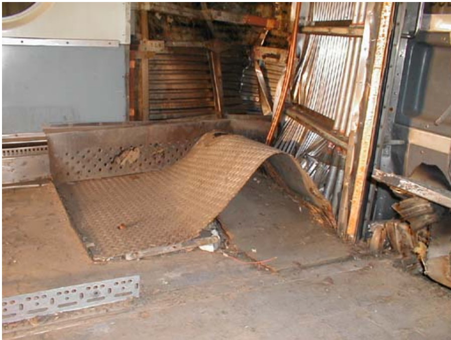
Figure B3-19. Left-side Floor Buckling Aft of Bulkhead Wall
