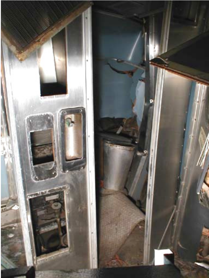
Figure B3-4. Inside View of Water Closet
