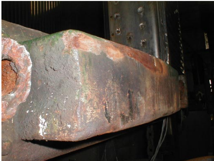
Figure B5-12. B-End Buff Stop—Collision Marks from Impact with Trailing Car
