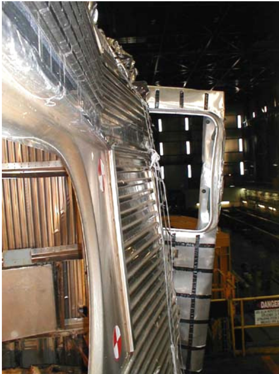
Figure B4-10. View of Right-side Superstructure from First Side Window, Looking Forward
