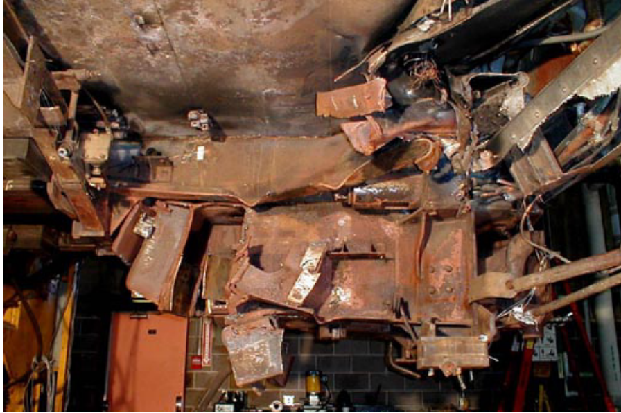
Figure B1-27. Right-side Draft Sill, From Side, After Non-Structural Material Removal
