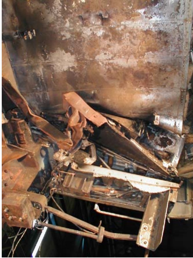
Figure B1-29. Forward Right-side Deformations - Buckling of the Floor Panels
