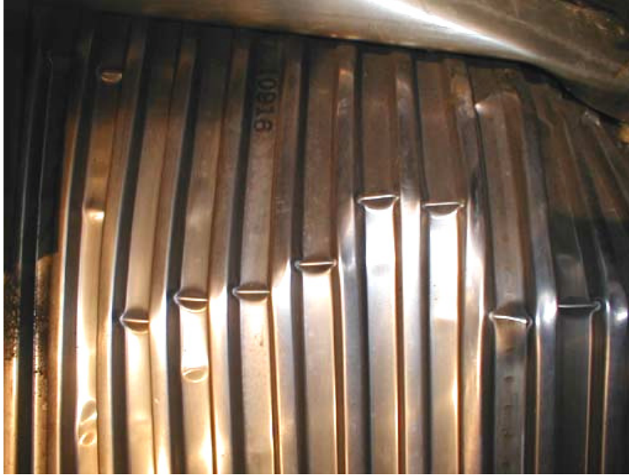
Figure B3-22. Skin Buckle on Upper Right-side of Bulkhead Wall—Typical Buckle Pattern of Superstructure Corrugated Skin
