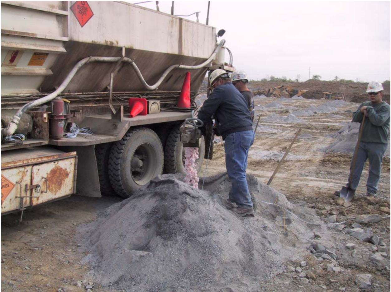
Figure 15 -- ANFO loaded into a borehole primed with a booster and Orica I-KON™ electronic detonator
