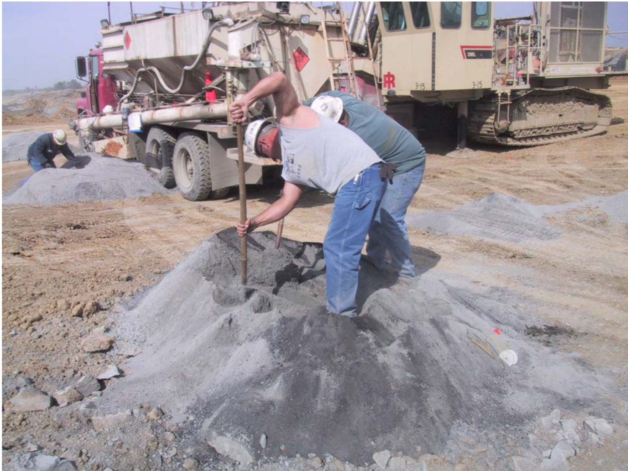
Figure 16 - Stemming the loaded blast hole
