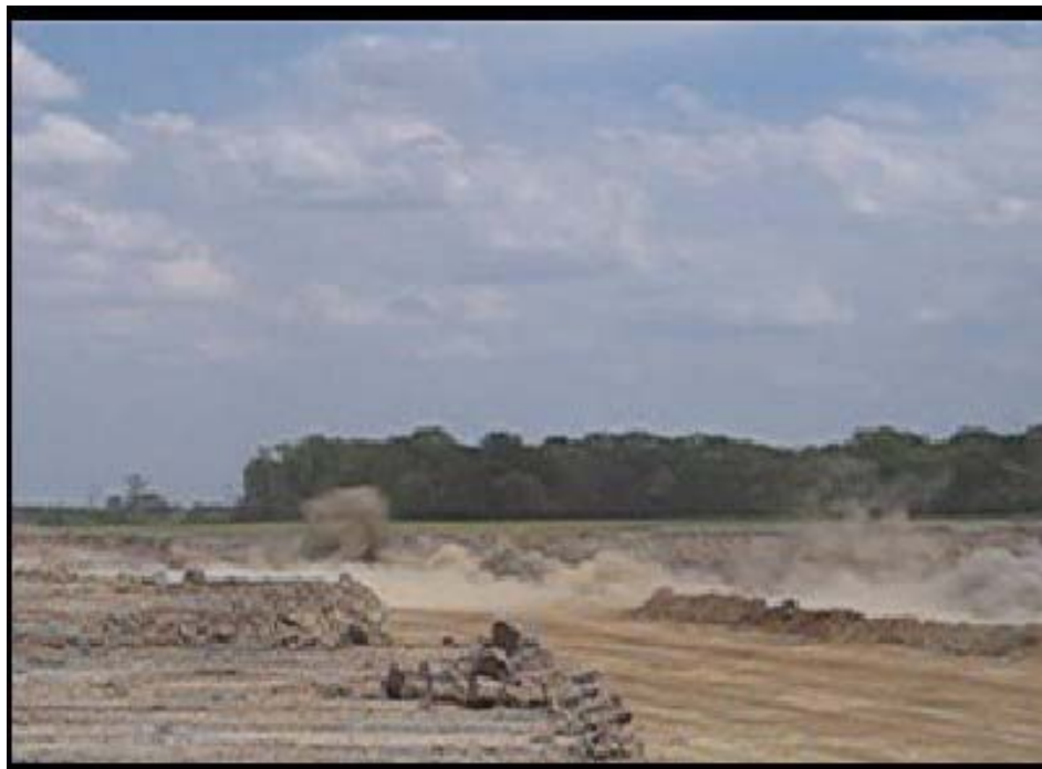
Figure 18 - Firing of a blast using the Orica I-KON™ electronic detonator system
