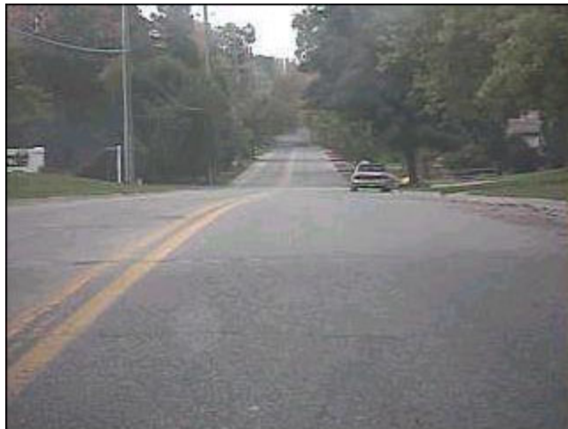
Figure 4.7 Unresolved Vertical Curvature
