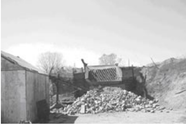
Figure 3: The skid steer loader traveled over the top of the grizzly and landed on the ground below
