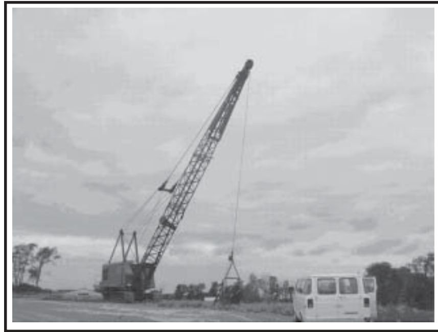
Manitowoc 3000 Crawler Dragline Crane
