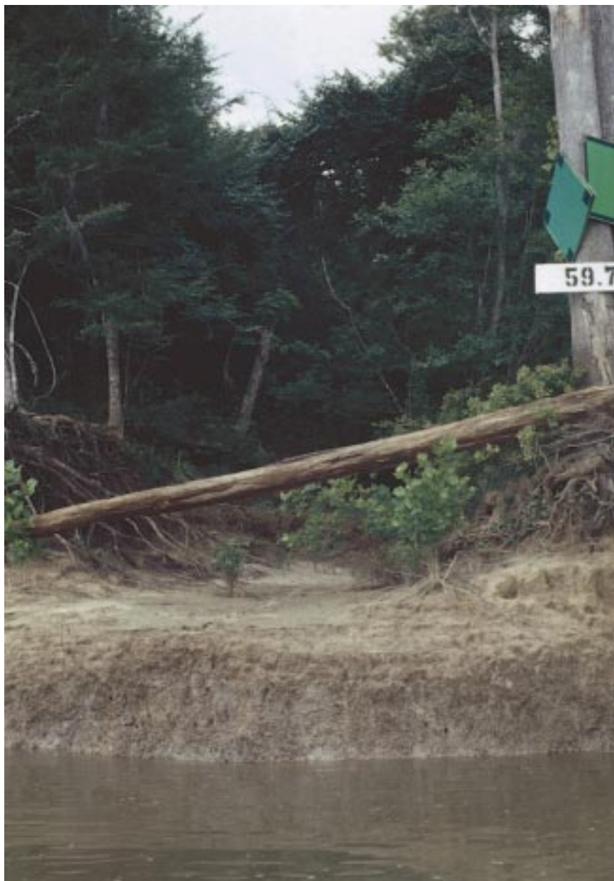
Figure 3. Example of general survey site with floodplain stream disconnected from the Apalachicola River at the time of observation. This unnamed stream at river mile 59.7 in the middle reach of the river had a streambed approximately 3.5 feet above the water level of the river when lagged flow was 9,600 cubic feet per second at the Chattahoochee gage. Using a stage-discharge rating representative of the middle reach of the river, the flow at the Chattahoochee gage at which this stream would be connected to the main channel was determined to be about 16,000 cubic feet per second.
