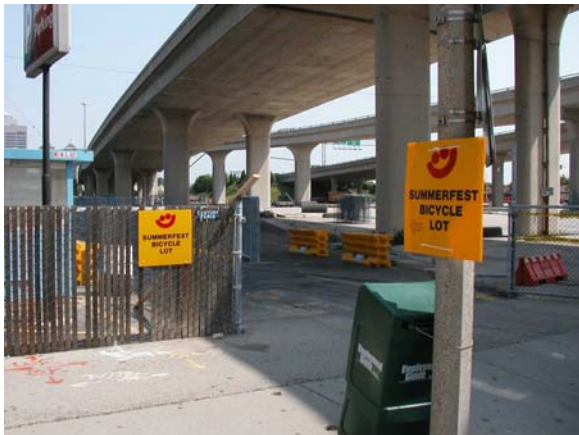
Figure 7-6 Bicycle Parking Area
