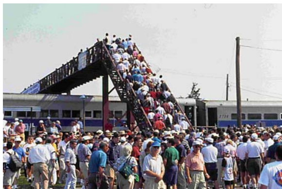
Figure 6-23 Temporary Pedestrian Bridge
