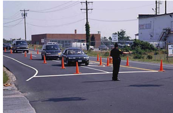
Figure 6-54 Positive Traffic Control
