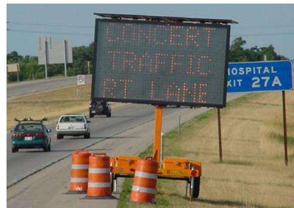
Figure 6-38 Portable Changeable Message Sign (Photo courtesy of the Wisconsin DOT.)
