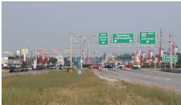
Figure 6-52 Road Block of Ingress Route to Facilitate Egress
