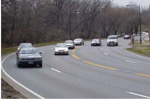
Figure 6-43 Daily Contraflow Operation
