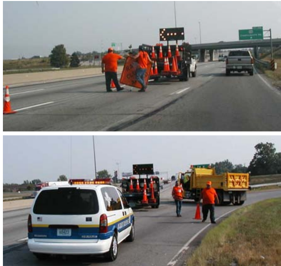
Figure 6-39 Temporary Elimination of Freeway Weaving Area
