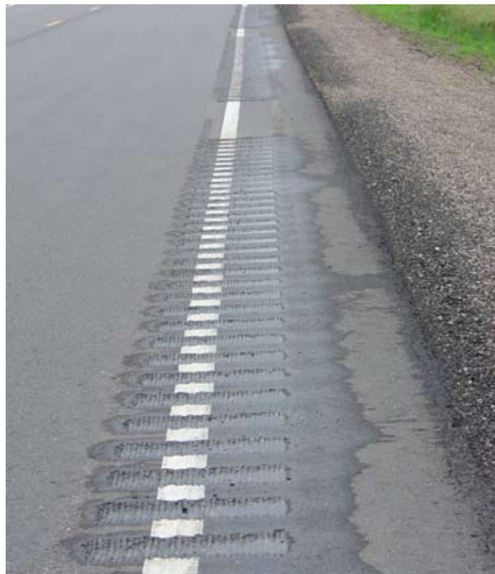
Figure 11. Rumble stripe during construction in Iowa. (Note: edge lines are repainted after rumble stripe cut.)
