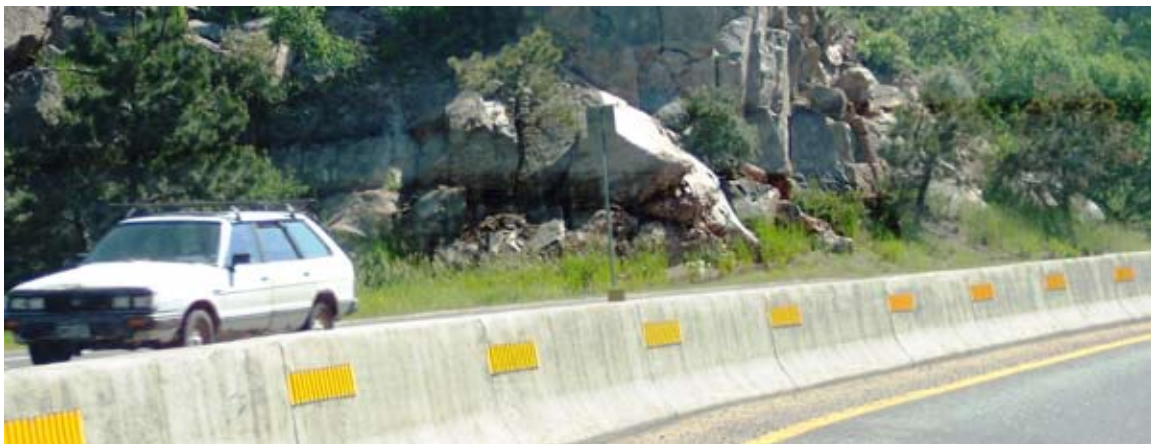
Figure 13. Sheet delineation on median barrier in Colorado.
