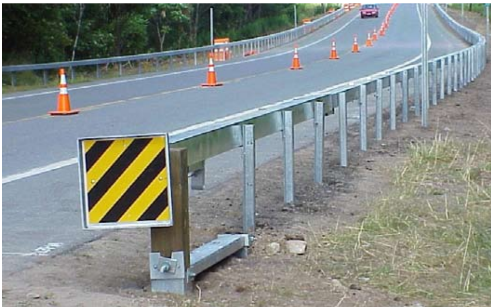
Figure 21. Box beam guardrail in New York. (Source: Courtesy of NYSDOT)
