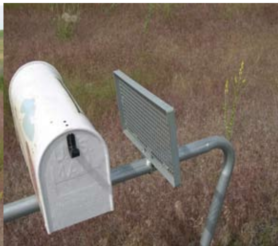
Figure 24. Close up of a crashworthy mailbox installation in Washington State.
