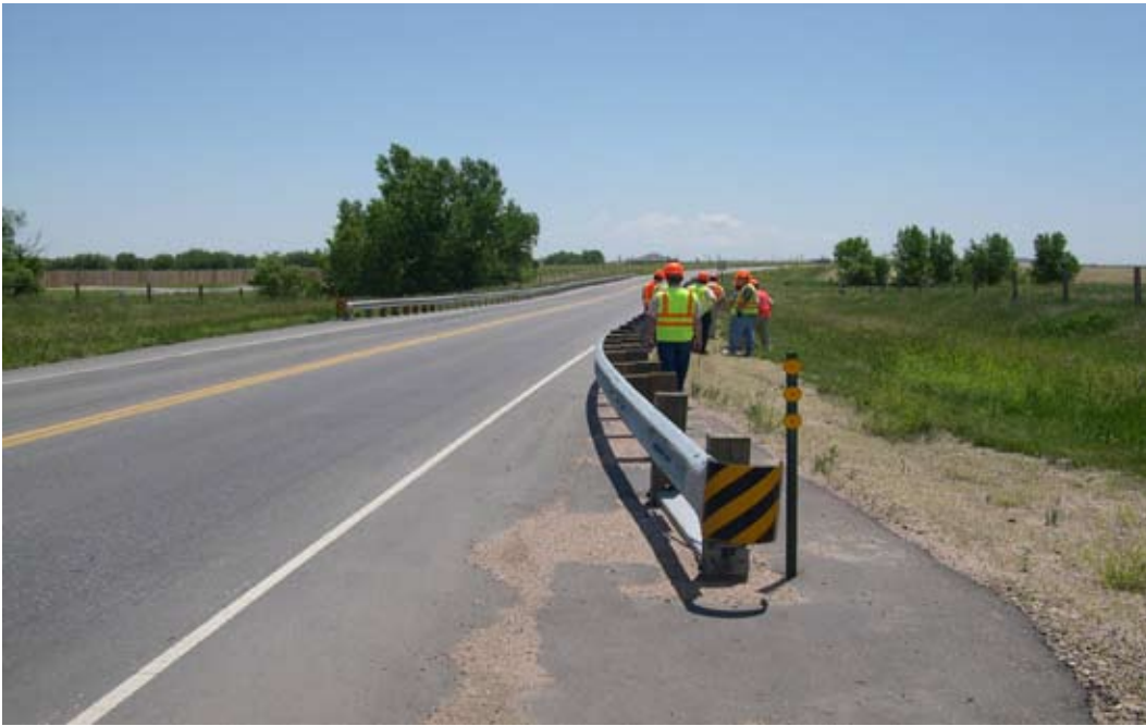
Figure 22. Guardrail terminal and pavement in Colorado.
