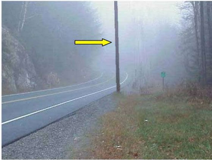
◀ Figure 25. Before utility pole relocation in New York. (Source: Courtesy of NYSDOT)
