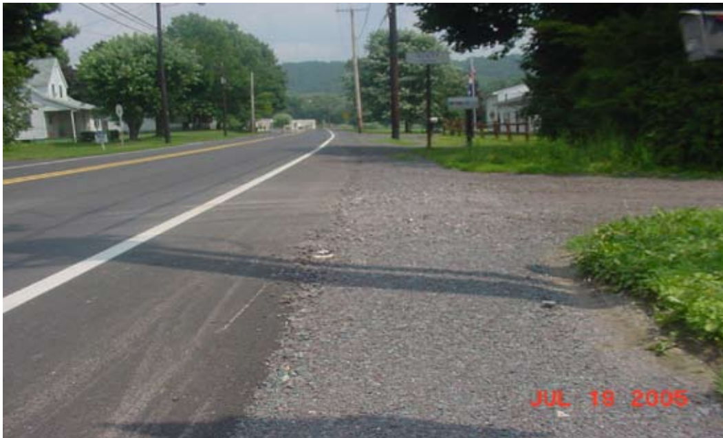
Figure 19. Full shoulder pavement with shoulder backup in Pennsylvania.
