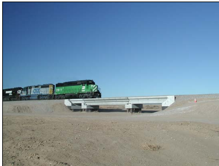
Figure 1. Test Train Over the State-of-the-Art Concrete Bridge at FAST
