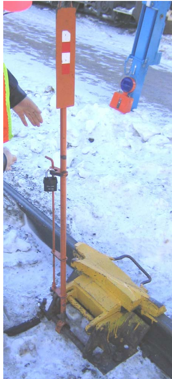
Figure 3. 5-Alive Requires Derails to be Positioned and Locked (This Derail has a Device to Keep the Lock Out of the Snow)
