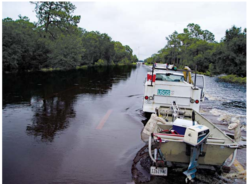
Figure 3 —View of road overflow at discharge of 9,900 ft 3 /s in Horse Creek near Arcadia (site 2, fig. 1, table 1) on June 23, 2003.
