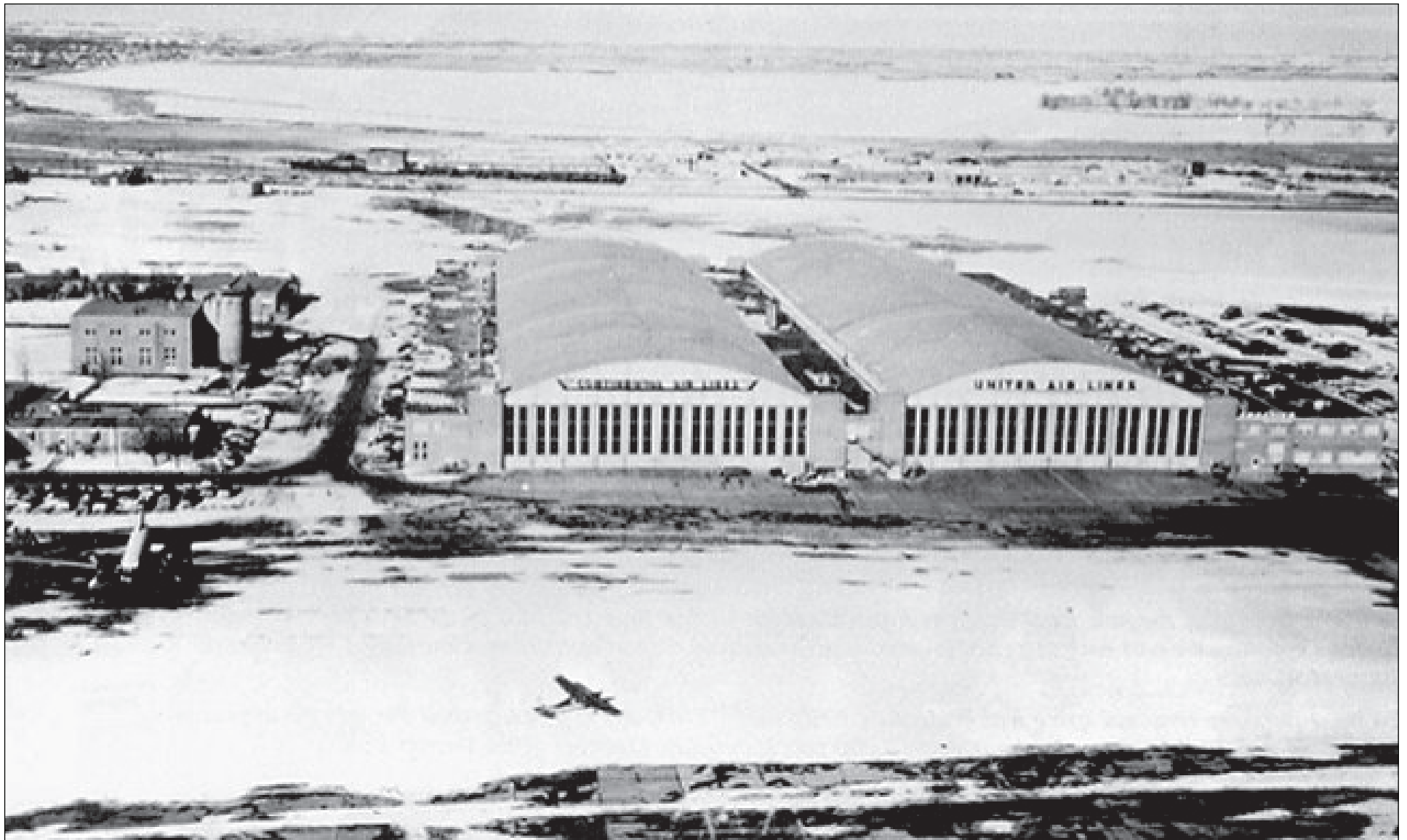
Figure 2-3: 1950s Photograph Showing Hangars 5 and 6
