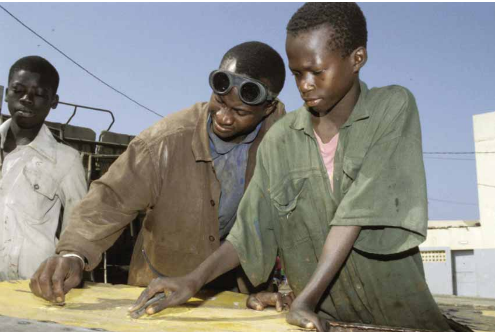
Teenagers working on a construction site. Senegal.
