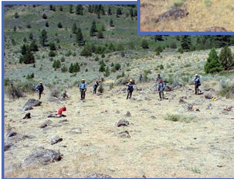
Section of fuel break after maintenance project.
