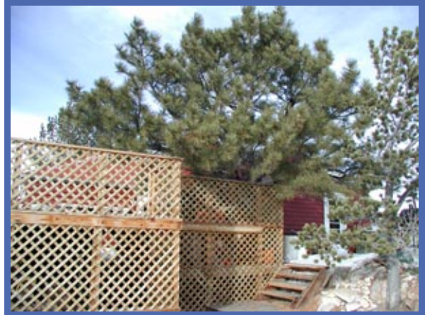
Deck built around tree creates risk.
