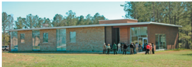
The Southern Regional Fire Training Center officially opened with a dedication ceremony on Tuesday, March 14, 2006.
