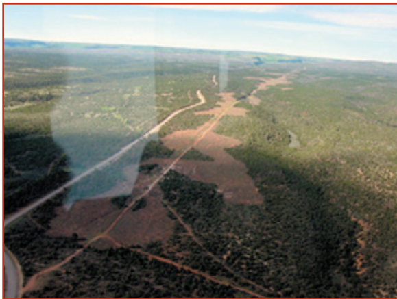
An aerial view facing southwest of the Highway 90 power line treatment.
